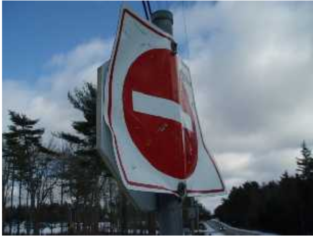
Typical aluminum traffic sign vandal damage caused by swinging from the sign – often occurs where students gather.
